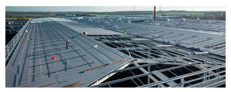
Recent fatalities during loading out and installing roof sheets on portal-framed structures has highlighted the need for improved guidance to help those writing method statements to protect their workers.
