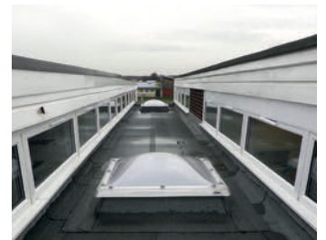
10 Rooflight Kerbs and Upstands
