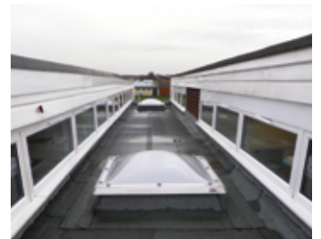
10 Rooflight Kerbs and Upstands
