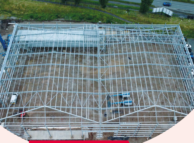
Figure 1: Portal-framed structure
