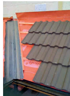
Tiles laid 'staggered' to valley
