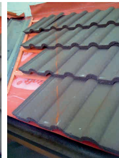
Line struck—two tile widths from desired finishing point in valley line
