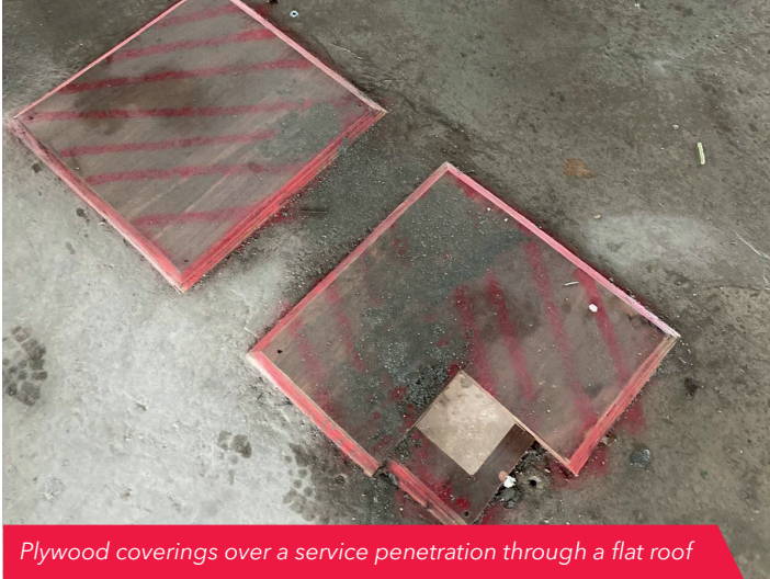
Example of a poorly covered hole
